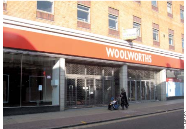
Former Woolworths Store, Peckham, London
